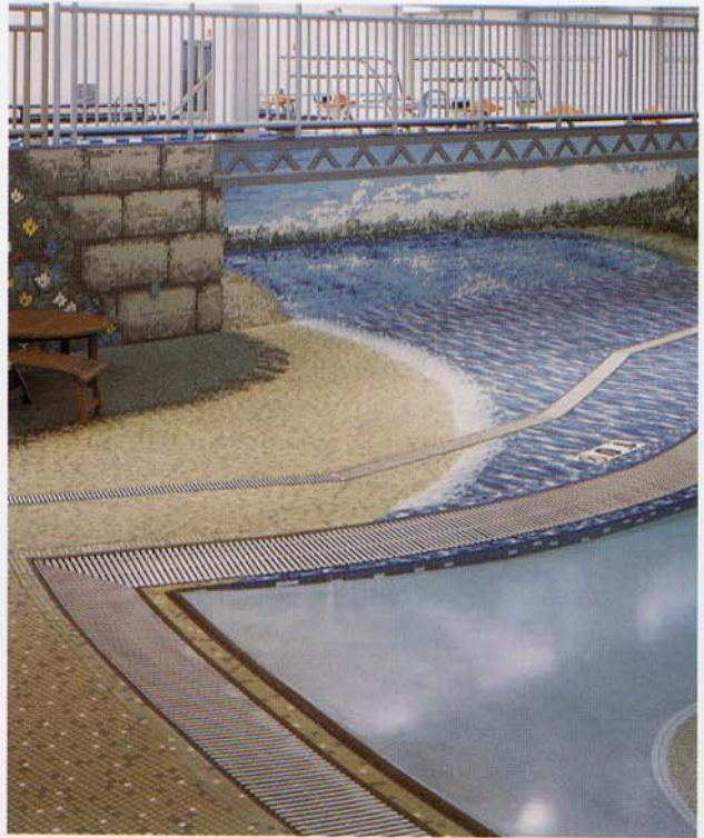
Westerville Community Center, Westerville, OH. Architect: John Poe Architects. Tile Contractor: Weiffenbach Tile and Marble Daltile Architectural Representative: Marsha McCauley. 1" x 1" Keystones mural.
