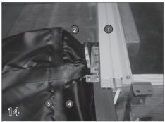
Pull the cover into the track so the leading edge loop is over the water.
