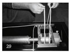
Tip: The rope for the non-motor side should be attached approximately 1-2 inches further down than the motor side rope depending on the width of the pool. Use the switch and operate the cover in the "Closed" position to cover the pool.
