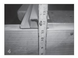
To attach the feet, first measure the distance from the bottom of the housing to the top of the track/encapsulation. (This will determine the height of the
