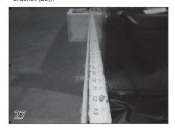
Leaving an extra 6-8 feet of extra rope length, pull on the ropes until the leading edge begins to move forward equally on both sides. Burn or wrap the rope with tape and cut to length.
