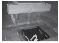
Installing The Cover Unroll the cover behind the housing from left to right. Unravel ropes to ensure there are no knots while running the rope
