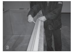
Pull the rope along the water side of the track towards the pulley end cap. Tip: Sometimes a guide feed can be put on to help feed the rope.
