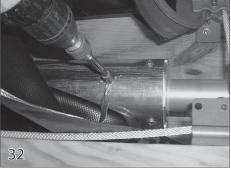
Using a self tapping screw (32), attach the bonding wire on both sides of the roll up tube.
