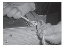
Wedge the rope into the inside rope channel of the track.
