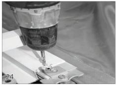
Drill through the center of the encapsulation and guide. Insert a 10-32 x 1 3/4 screw (42) and nylock nut (29). This step is very important. This will prevent the guide from sliding into the cover housing duirng the operation of the cover system.
